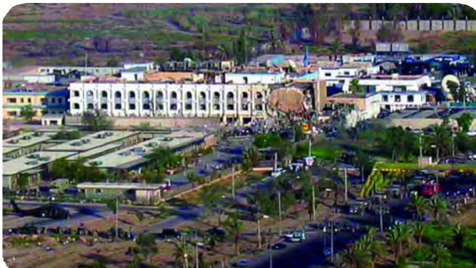
Damaged area of UN HQ facility in Baghdad.
